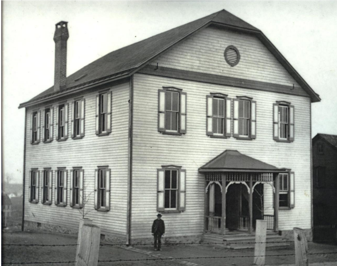
The "new" schoolhouse located on Pine Street
